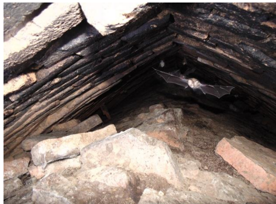
Fig-25, Vaulted roof of eastern vestibule in the ground floor is visible through the small hole
