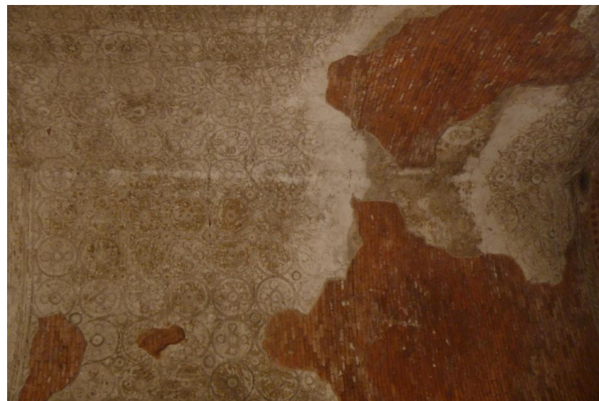
Fig-30, Roof of the vestibule of the Htilominlo Temple
