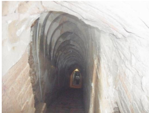
Fig-11, Stair-case of the ground floor
