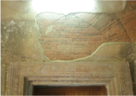
Fig-36, Radiating arch above the straight arch
