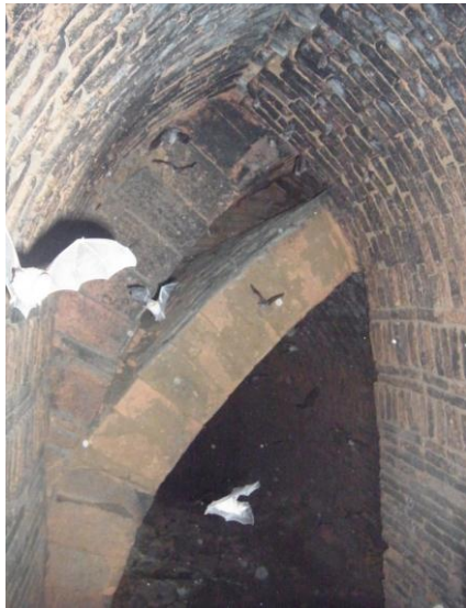
Fig-29, Semi-circular double-layered lean-to-vault inside the secret entresol
