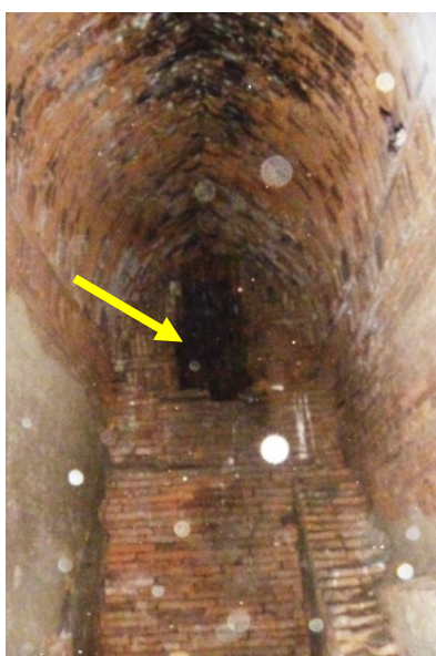
Fig-19, Small hole (Southern entrance)
