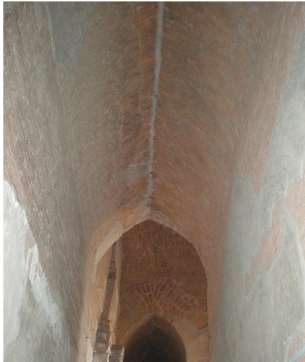
Fig-34, Tunnel vault, Roof of the corridor
