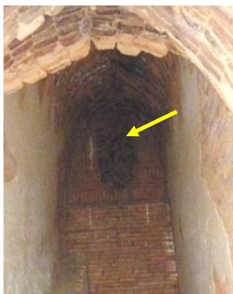
Fig-20, Small hole (Northern entrance)
