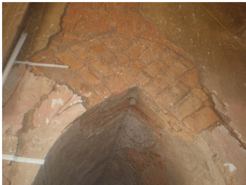
Fig-35, Three-layered radiating arches inside the corridor
