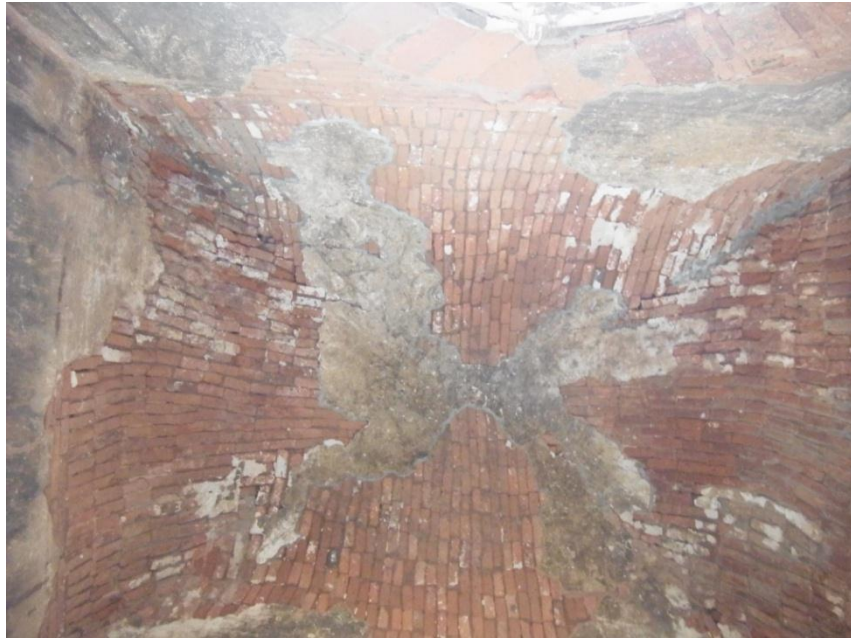
Fig-31, Roof of the Gate-way
