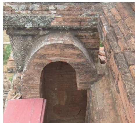
Fig-43(c), Decorative brick art works in the roof of stair-cases
