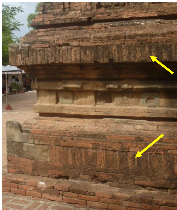
Fig-41, Vertically bricks alignments supported to the curvilinear roof
