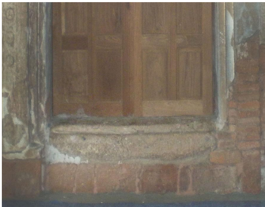
Fig-9, Sandstone threshold at the lower frame of the small room
