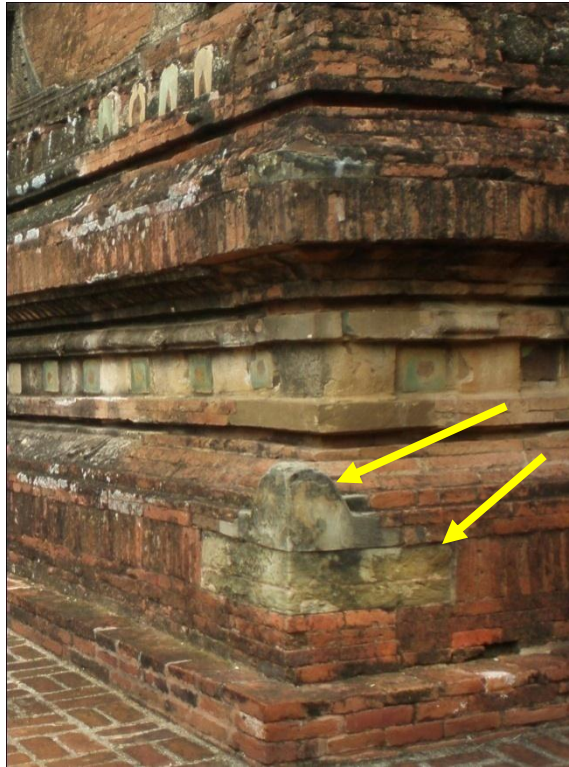
Fig-2, Corner sandstone of the GonNyinHtaung and carved sandstone dadoes above it
