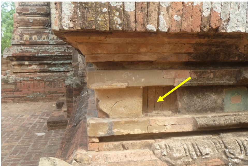
Fig-40, Vertically bricks alignment on which covered with glazed sandstone slabs
