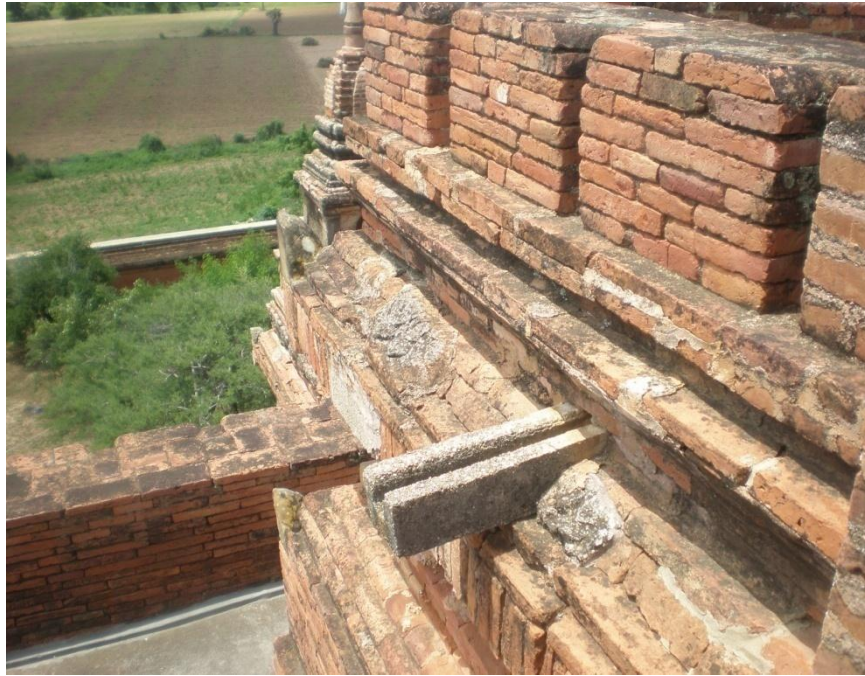
Fig-6, Sandstone drain-pipe
