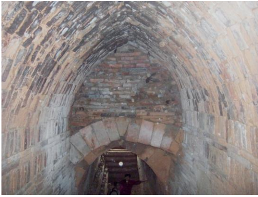
Fig-27, Radiating arch inside the long cave
