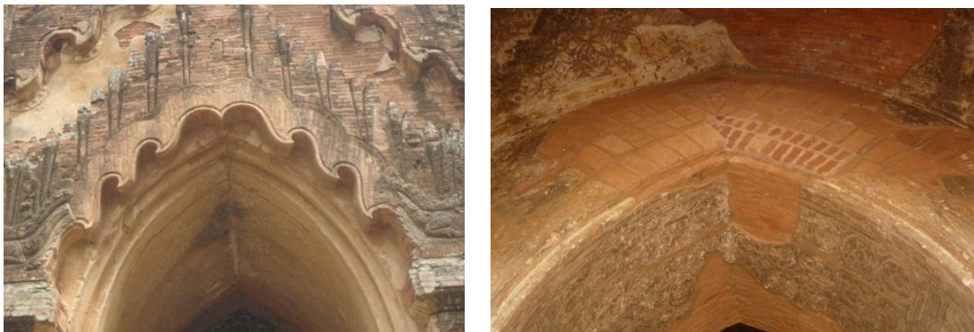
Fig-32, Three-layered radiating arch at the vestibule
