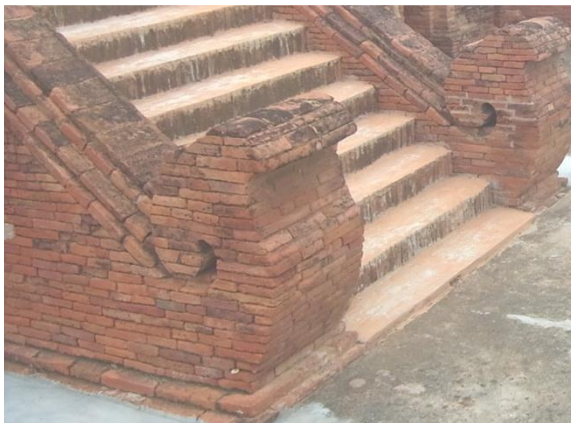
Fig-43(b), Decorative brick art works in the head of stair-cases as the shape of young mangoes fruits
